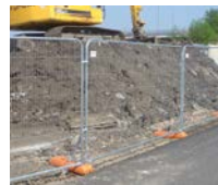
Site Security Fence Panels
